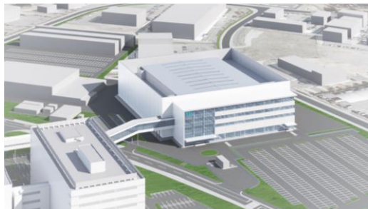
Koshi-city, Kumamoto Prefecture Completion scheduled for summer 2025
