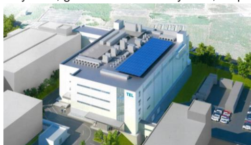
Nirasaki City, Yamanashi Prefecture: approx. ¥11.0B construction cost (Completion scheduled for Spring 2023)
