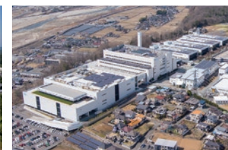
Tokyo Electron Technology Solutions Yamanashi Office Production Building Began operations in August 2020
