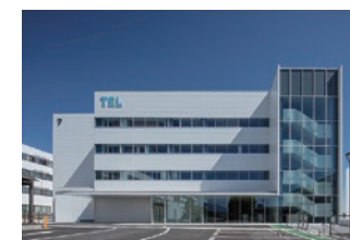
Tokyo Electron Technology Solutions Hosaka Office New Development Building (Completed in July 2023)
