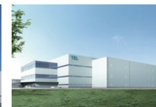
Tokyo Electron Miyagi New Development Building (Completion scheduled for spring 2025)
