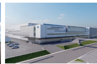
Tokyo Electron Technology Solutions Tohoku Office Tohoku Production and Logistics Center (provisional name) Completion scheduled for autumn 2025
