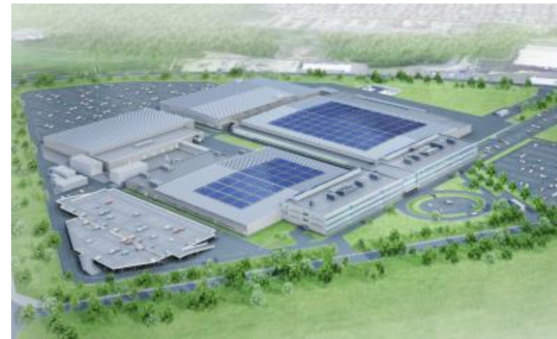
Tokyo Electron Miyagi's new development and logistics buildings
