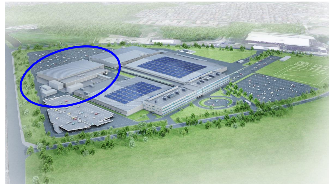
Tokyo Electron Miyagi Ltd. New development building and logistics building
